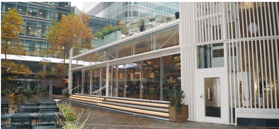
The Oasis Bar building sits in an elevated position which allows the pipes from the Sanicom 2 to run under the ground to the soil and vent pipe in the external customer WCs.
