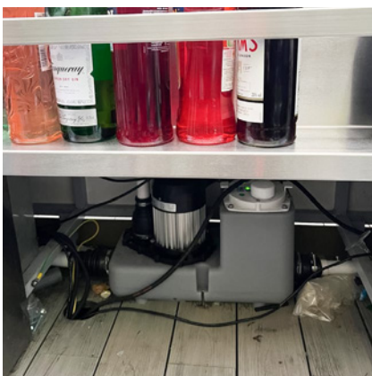
The Sanicom 1 takes waste from the upstairs bar and discharges it to the same SVP as the Sanicom 2.
