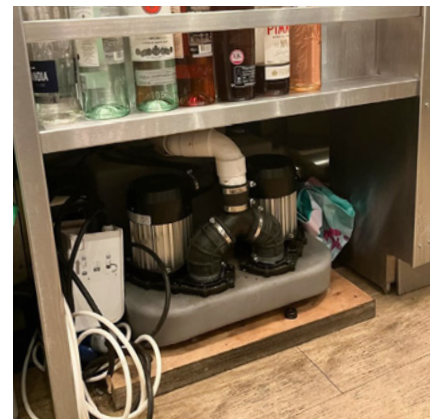
The Sanicom 2 features twin pumps to ensure continuity of service.
